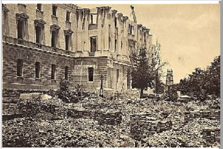
The unfinished State House ( Note Trinity Cathedral )
